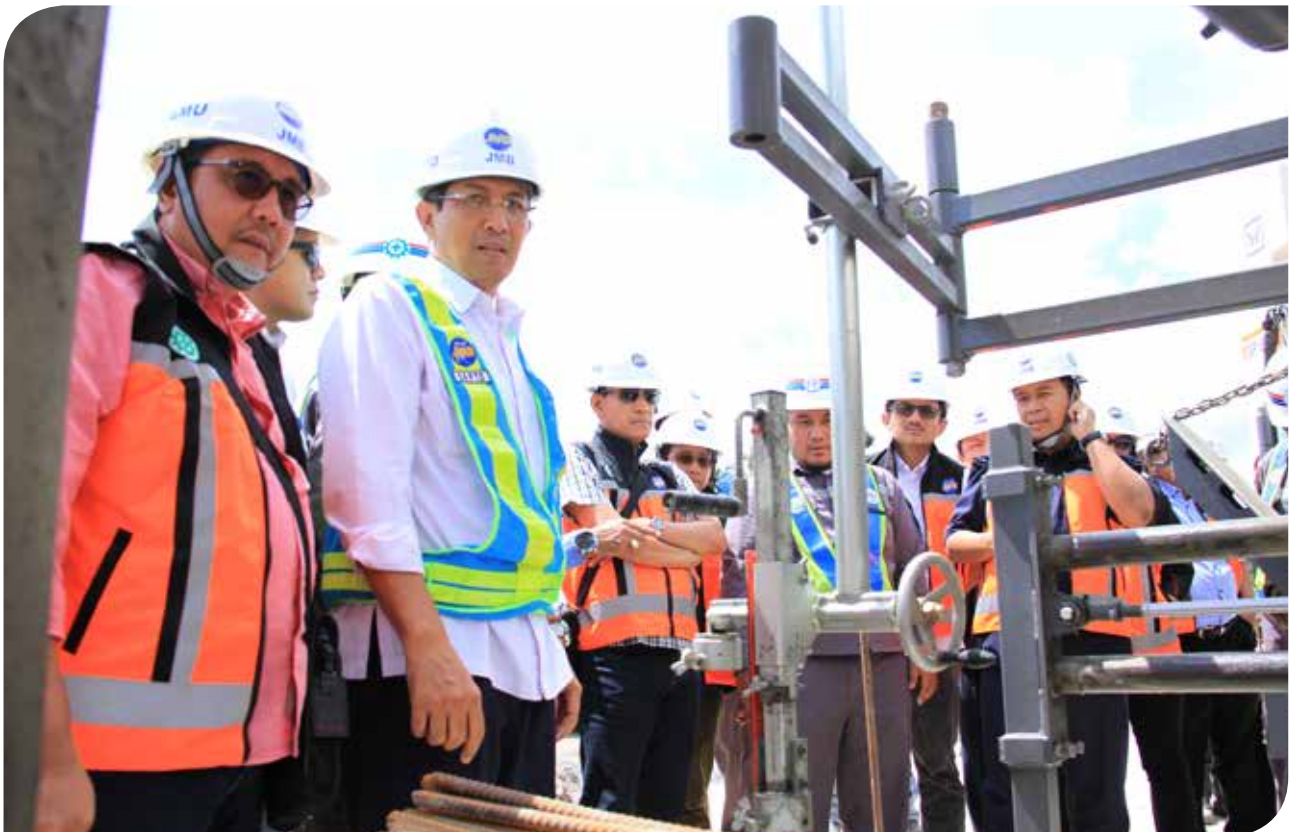
The visit of Board of Commissioners to Balikpapan-Samarinda Toll Road Project.
