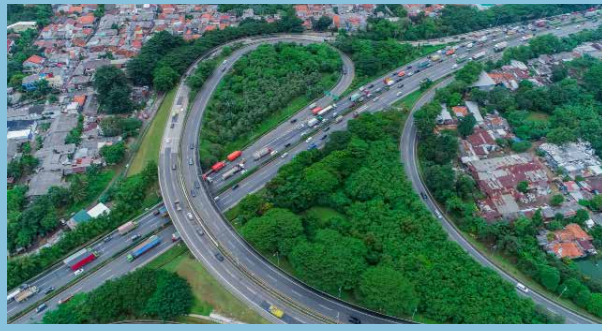
Kategori Penghargaan Jalan Tol Panjang 15 - 50 KM Ruas Jalan Tol JORR non S - Peringkat 3 Award Category for Toll Road Length 15-50 KM JORR NON S Toll Road Section – 3rd place
